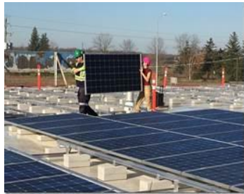
*SSC Crew Rooftop Installation
